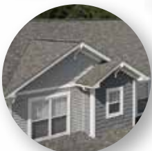
Roofing and Ventilation
